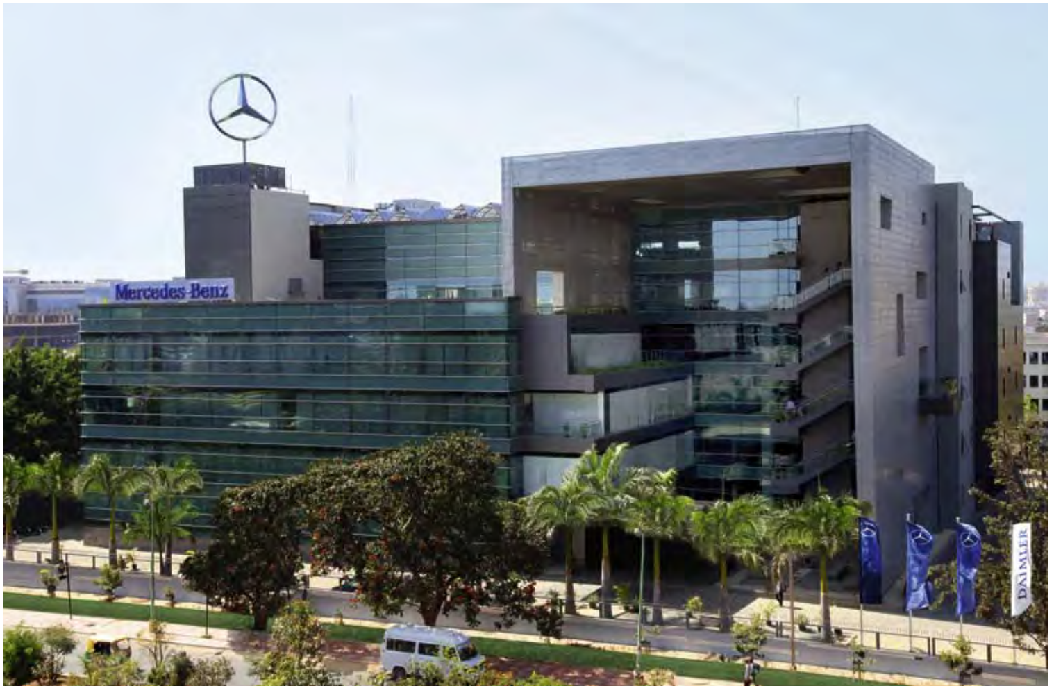
The biggest research and development location outside Germany – and part of our global growth strategy: the newly opened Mercedes-Benz Research and Development Center India in Bangalore.
